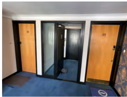
Double door fire lobby onto the central stairs.
