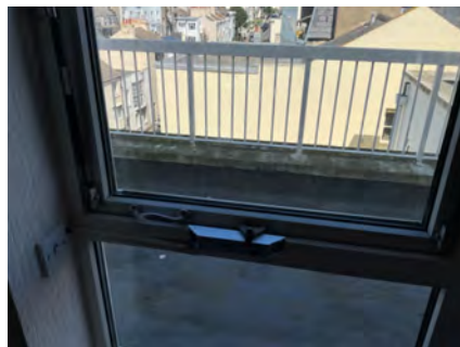
Example of AOV 5th floor.
