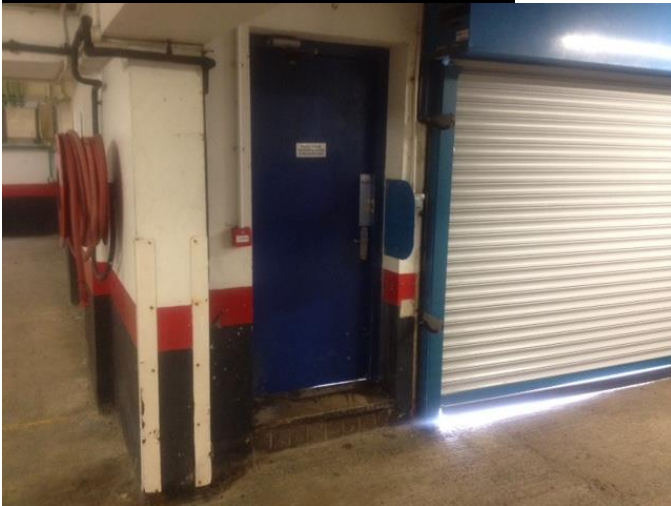
Left of Garage door exit
